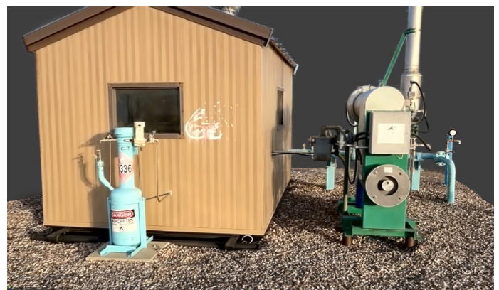
Figure 5. 3DGS rendering of an industrial scene showing photorealistic reconstruction of reflective surfaces, glass, cables, and piping from smartphone video.
